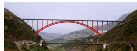
Fig. 2. Fengjie Meixihe Bridge (Reprinted with permission from Mr. Tingmin Mou)
