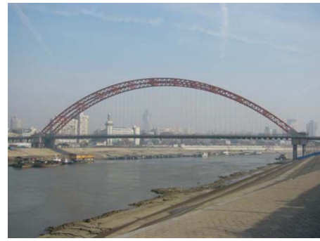
Fig. 6. No. 3 Hanjiang Bridge (Reprinted with permission from Ms. Ye Sheng)
